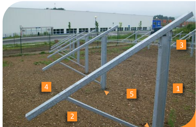
EASY TRACK WITH A 25 OR 30 DEGREE SLOPE OF THE MODULE CONSISTING OF THE RIGHT-ANGLED BAR, THE IPE 120 SUPPORTS, AND SLANTED BRACES
