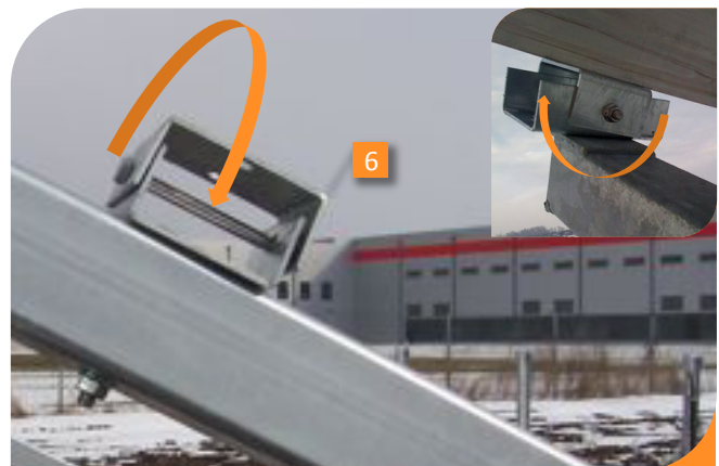
EASY TRACK WITH A 25 OR 30 DEGREE SLOPE OF THE MODULE CONSISTING OF THE RIGHT-ANGLED BAR, THE IPE 120 SUPPORTS, AND SLANTED BRACES
